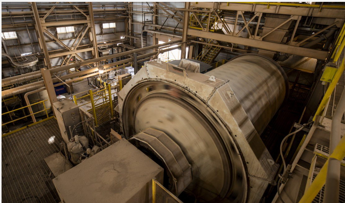
A ball mill turns during processing at the Mountain Pass mine in California. America's only rare earths producer exports all its output to China. Photo: Bloomberg
